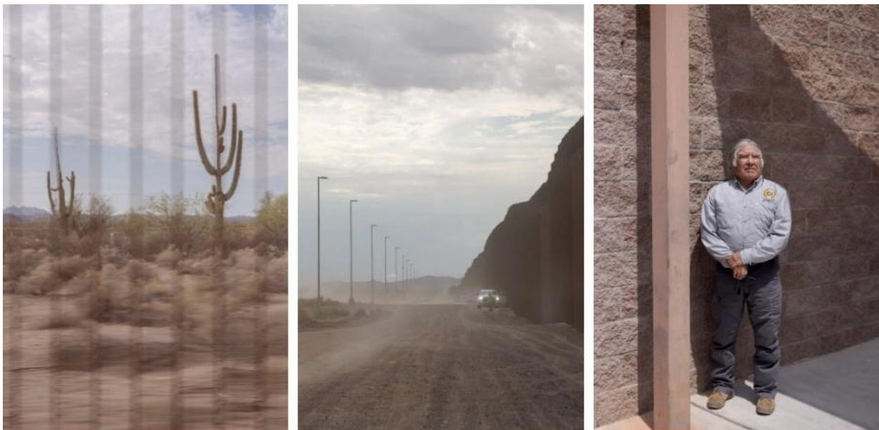
The border wall now under construction in Organ Pipe National Monument outside of Ajo, Ariz. Samuel Fayuant, a cultural affairs specialist with the tribe, is seen in the third photo above.
