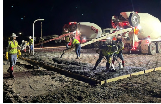
Pouring concrete for the Charco basketball court.
