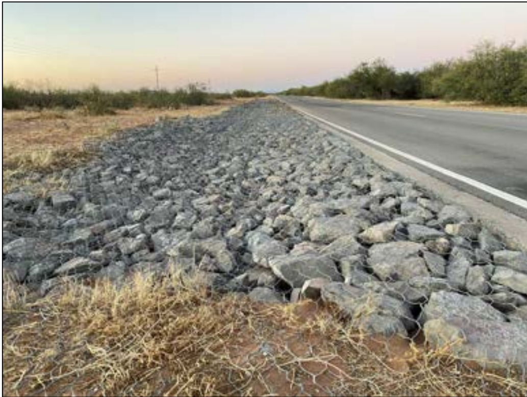
Roadside gabion baskets and refreshed pavement
