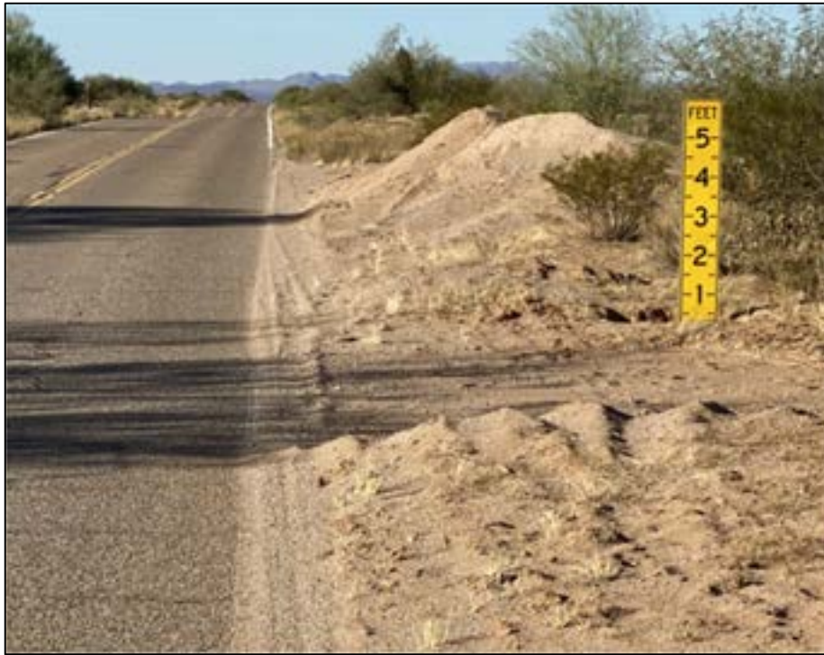
Example of depth gauges at road wash crossings
