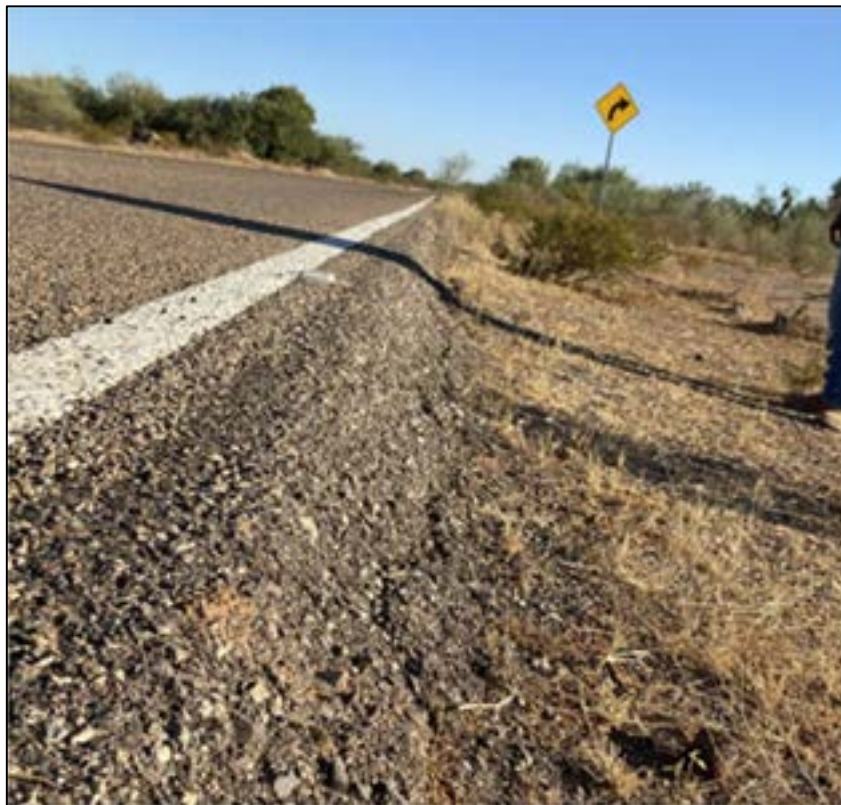
Typical pavement edge drop-off on Route 21
