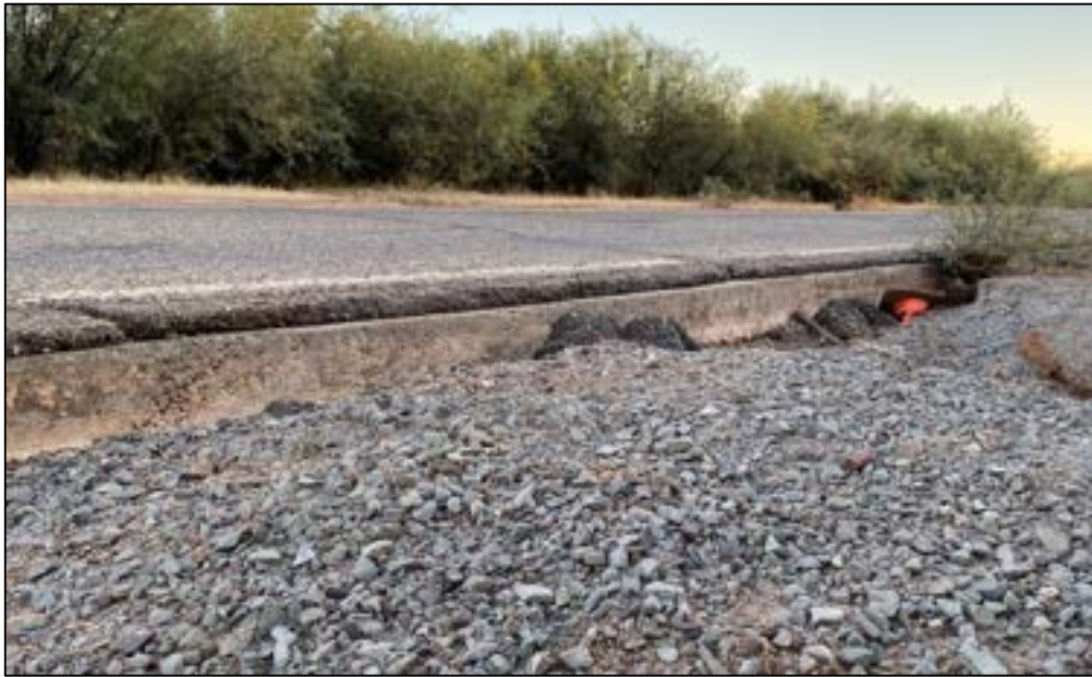
Large pavement edge drop-off on Route 21
