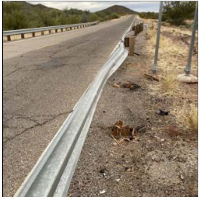
Existing damaged guard rails at mile markers 25.5, 20.5, 19, and 9.5 on route 19
