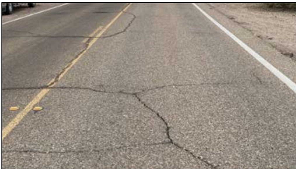
Cracking and pitting on Route 19
