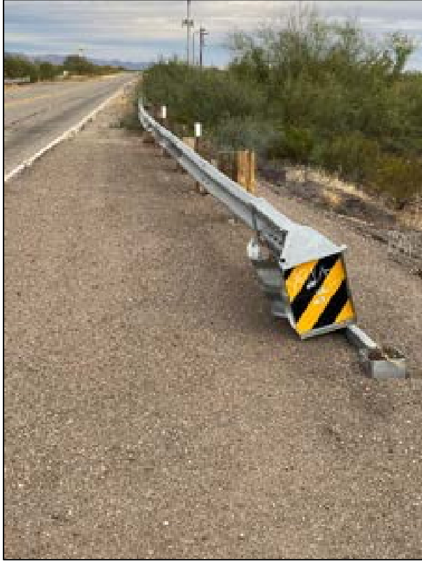
Existing damaged guard rails at mile markers 25.5, 20.5, 19, and 9.5 on route 19
