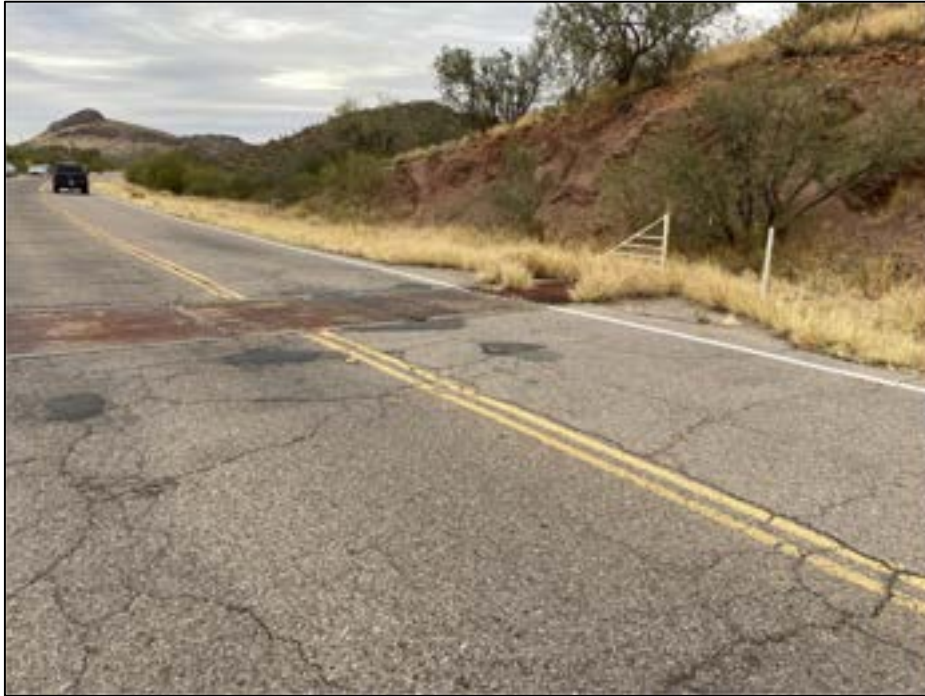
Existing cattle guard in the curve at mile marker 23.5 on route 19
