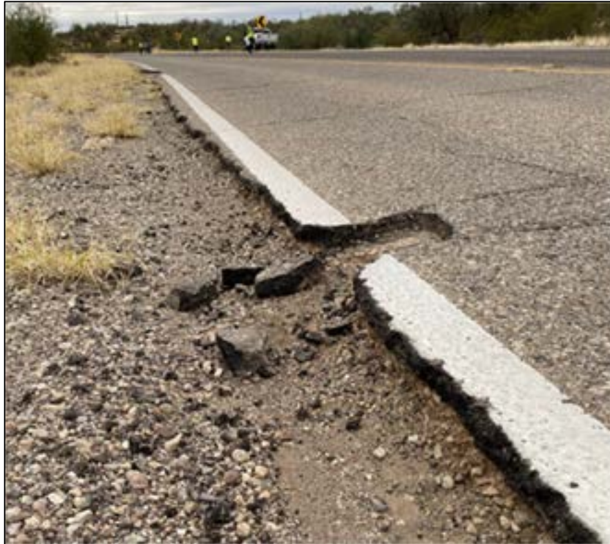
Pavement potholes and cracking on the shoulder of Route 19
