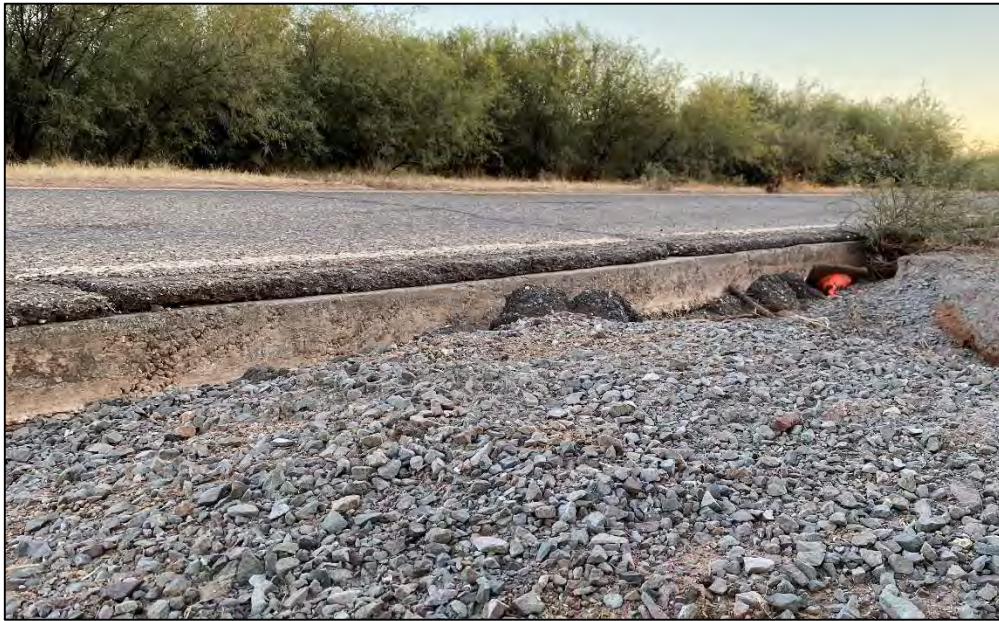
Large pavement edge drop-off on Route 21
