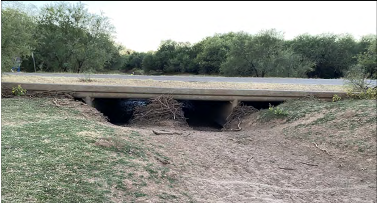
Clogged and blocked 5 span box culverts under Route 21
