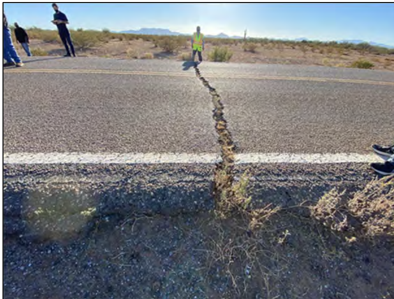
Pavement damage on Route 21
