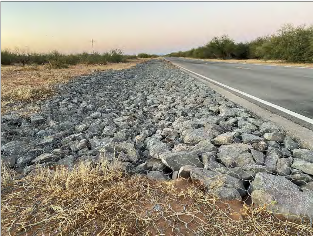
Roadside gabion baskets and refreshed pavement
