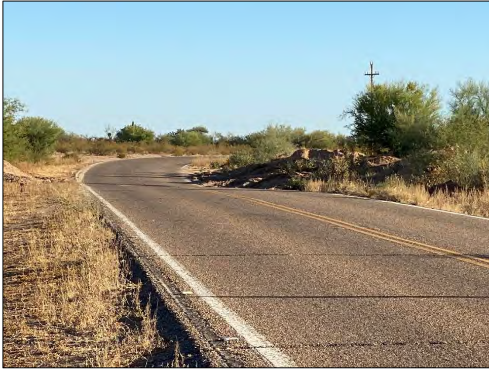
Example of existing road curve with a lack of delineation/chevrons
