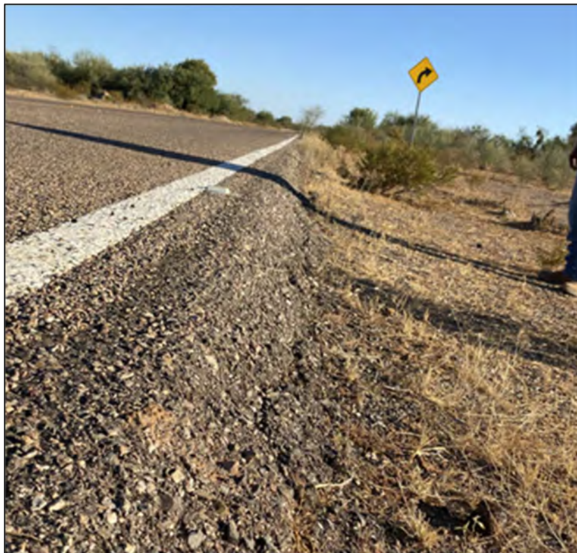
Typical pavement edge drop-off on Route 21
