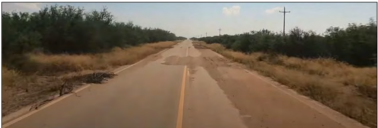
Soil accumulation on Route 21 at mile marker 11
