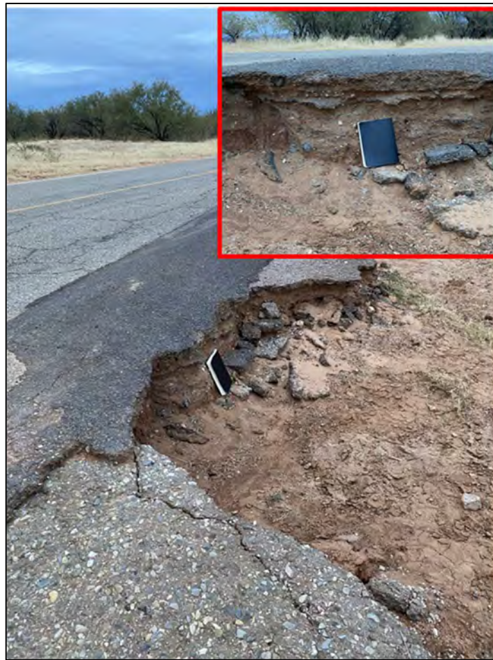
Sub road soil erosion at mile marker 18.25 on Route 19
