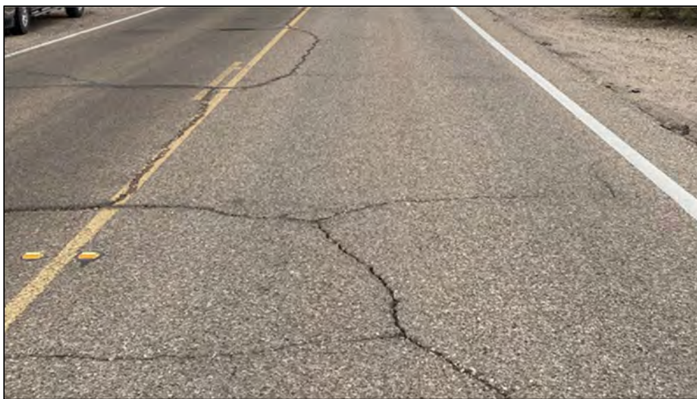
Cracking and pitting on Route 19
