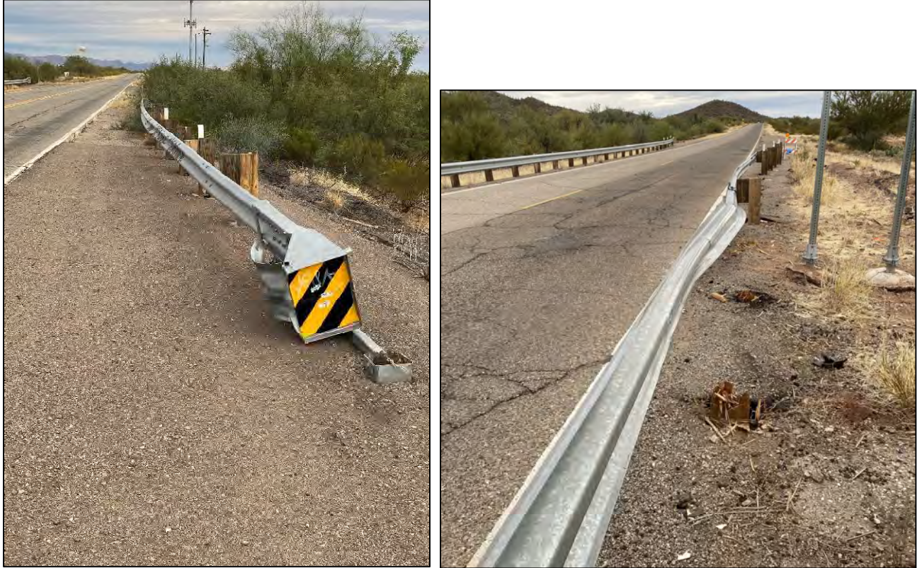
Existing damaged guard rails at mile markers 25.5, 20.5, 19, and 9.5 on route 19
