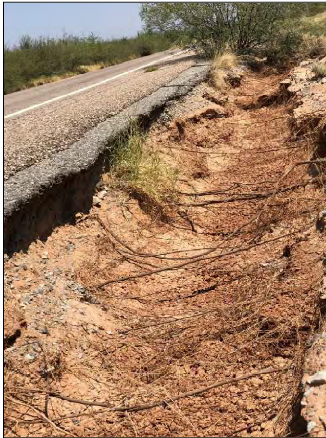
Extensive shoulder and sub-roadway erosion, as reported by Rita Wilson.
